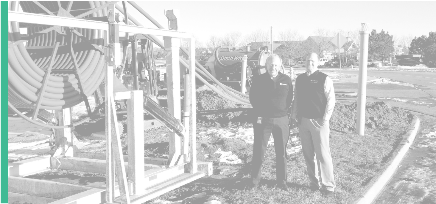
Construction of fiber backbone in Centennial, CO.
