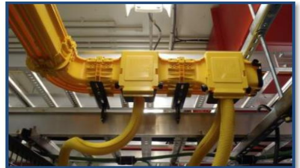
Figure 5-2: ADC Fiber System
